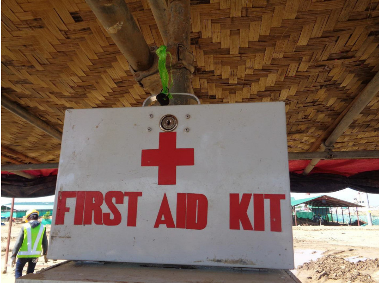
Photo No. 12. First Aid station at the Project construction site
