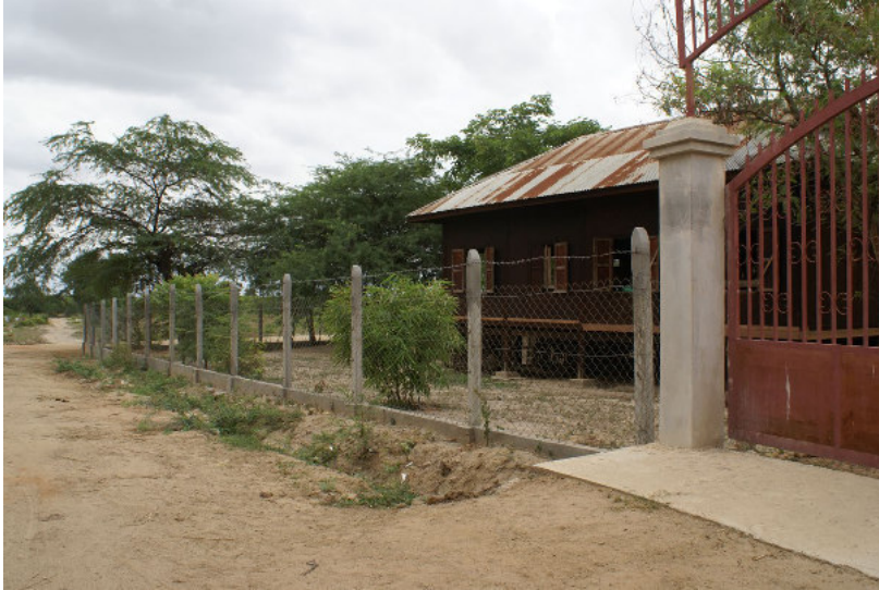
New fence at the school
