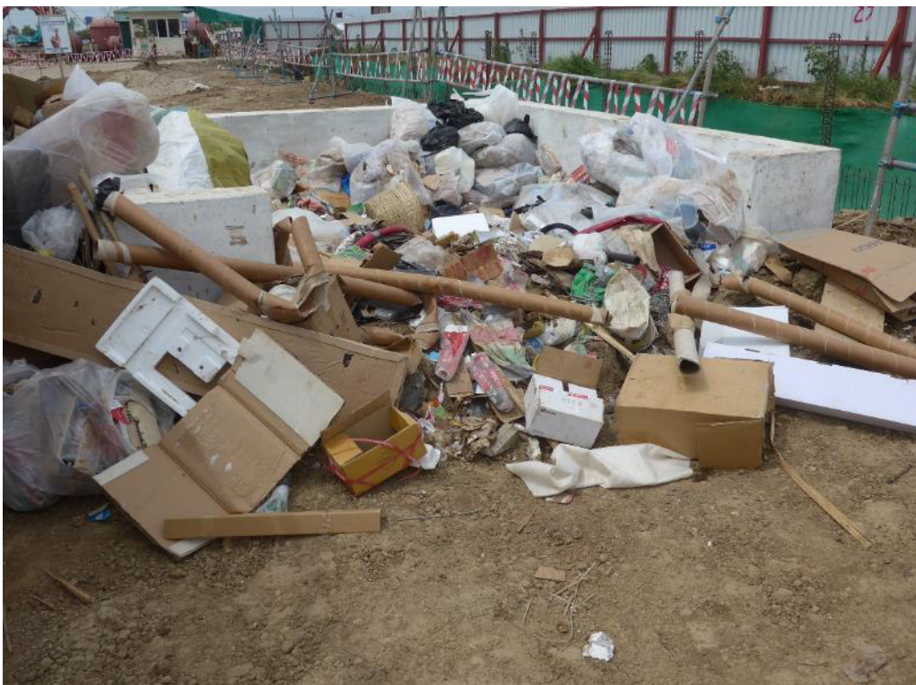
Photo 18: Inadequate containment of general waste
