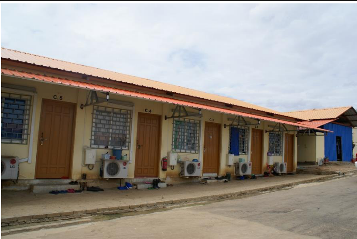
Photo 32: New zinc roof with drainage at JEM workers camp
