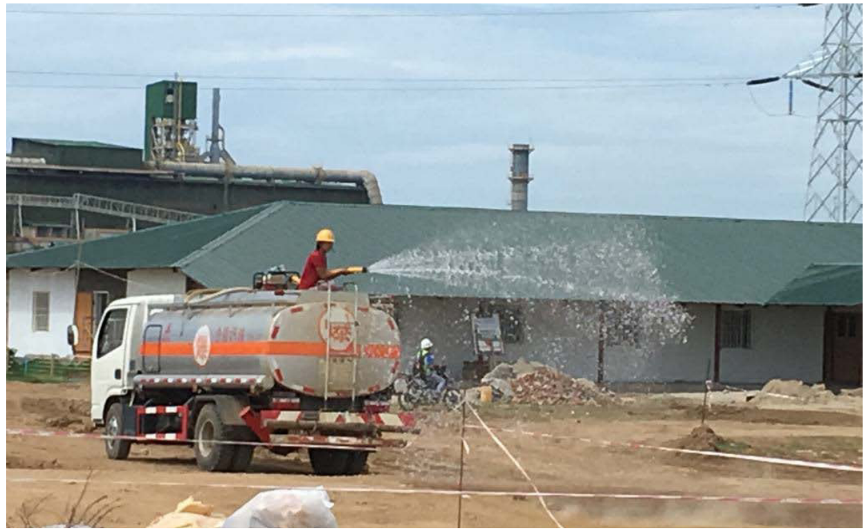
Photo 3: Dust suppression on site roads
