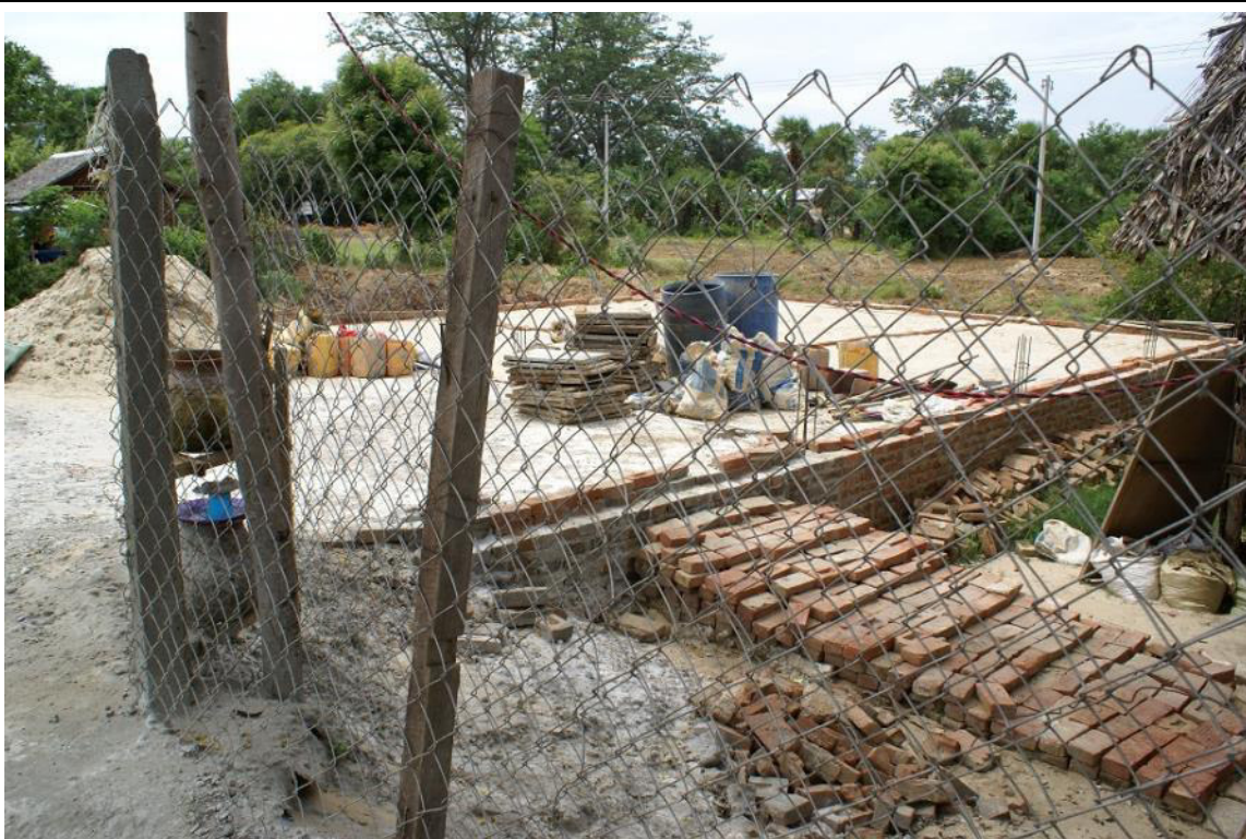
Photo 42: Foundation for new house built with farmer's crop compensation
