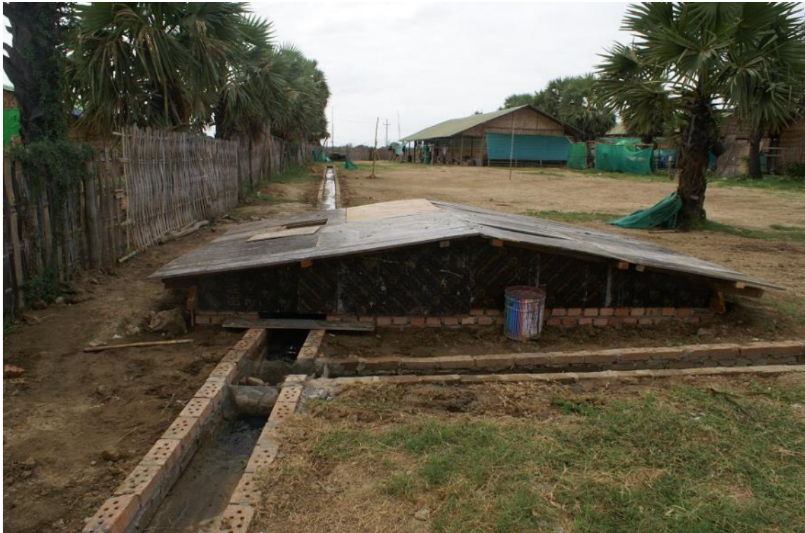
Photo 29: New drainage storage tank at Min Dhama camp
