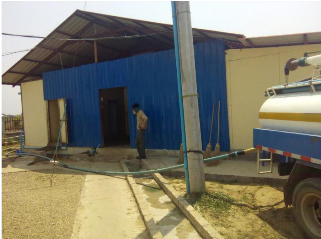
Photo 5: Vacuum tanker collecting sewage from septic tank at JEM camp
