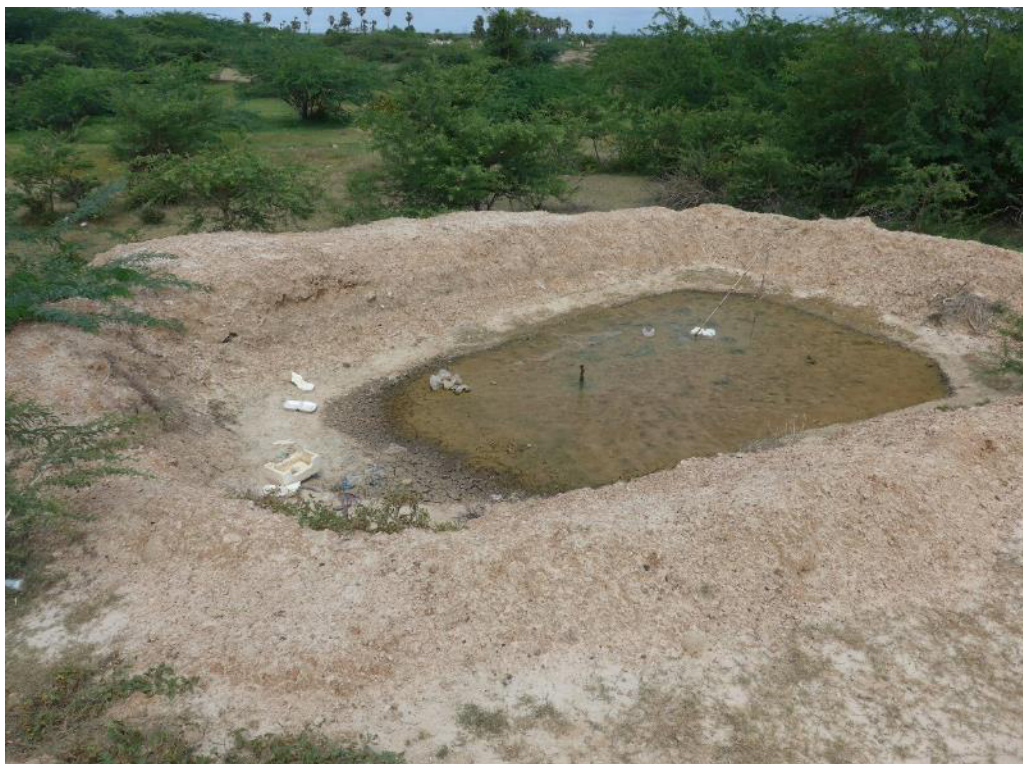
Photo 6: Wastewater disposal pit, reportedly used for disposal of sanitary wastewater
