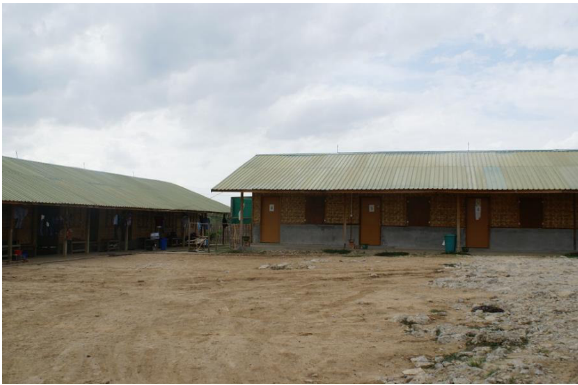
Photo 37: New zinc roof at the Min Dhama workers camp
