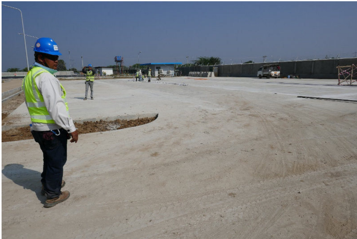
Photo 21: Car park outside Administration Building
