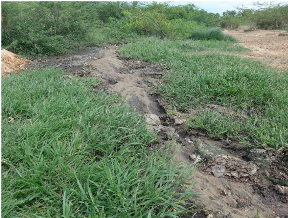
Photo 17: Evidence of wastewater disposal on soil adjacent to pit
