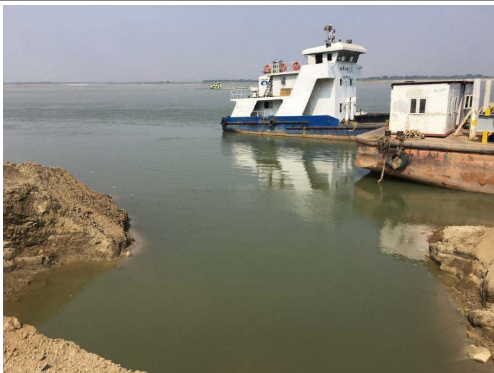
Photo 4: Nyaung Hla “jetty”, which is no longer used by the Project
