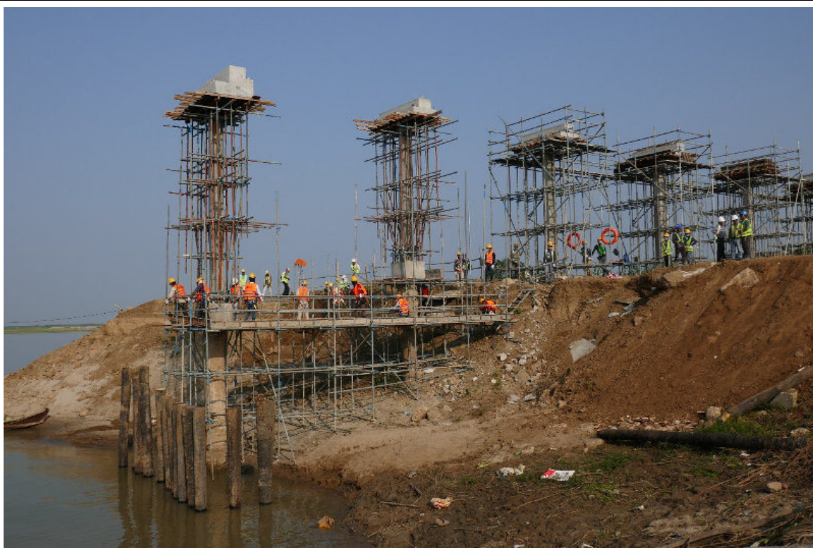
Photo 2: Final section of river water supply pipeline
