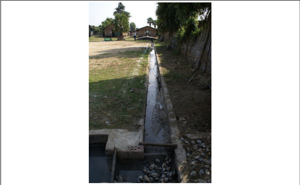
Photo 37: Well-maintained drainage system at the Min Dhama workers' camp
