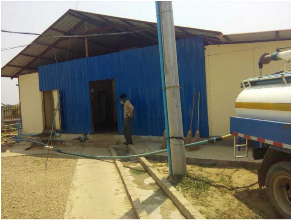
Photo 15: Vacuum tanker collecting sewage from septic tank at JEM camp
