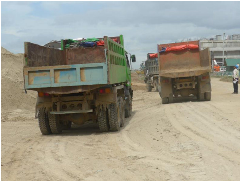
Photo 8: Trucks fitted with covers that are used when conveying soil and dusty materials
