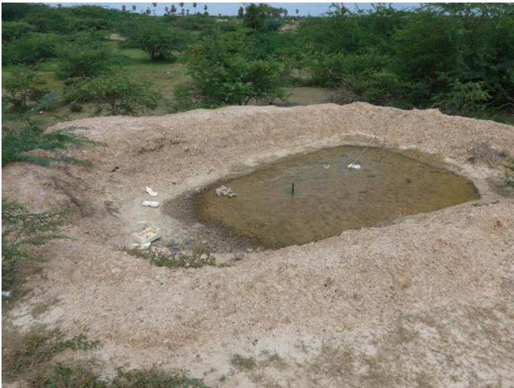
Photo 16: Wastewater disposal pit, reportedly used for disposal of sanitary wastewater
