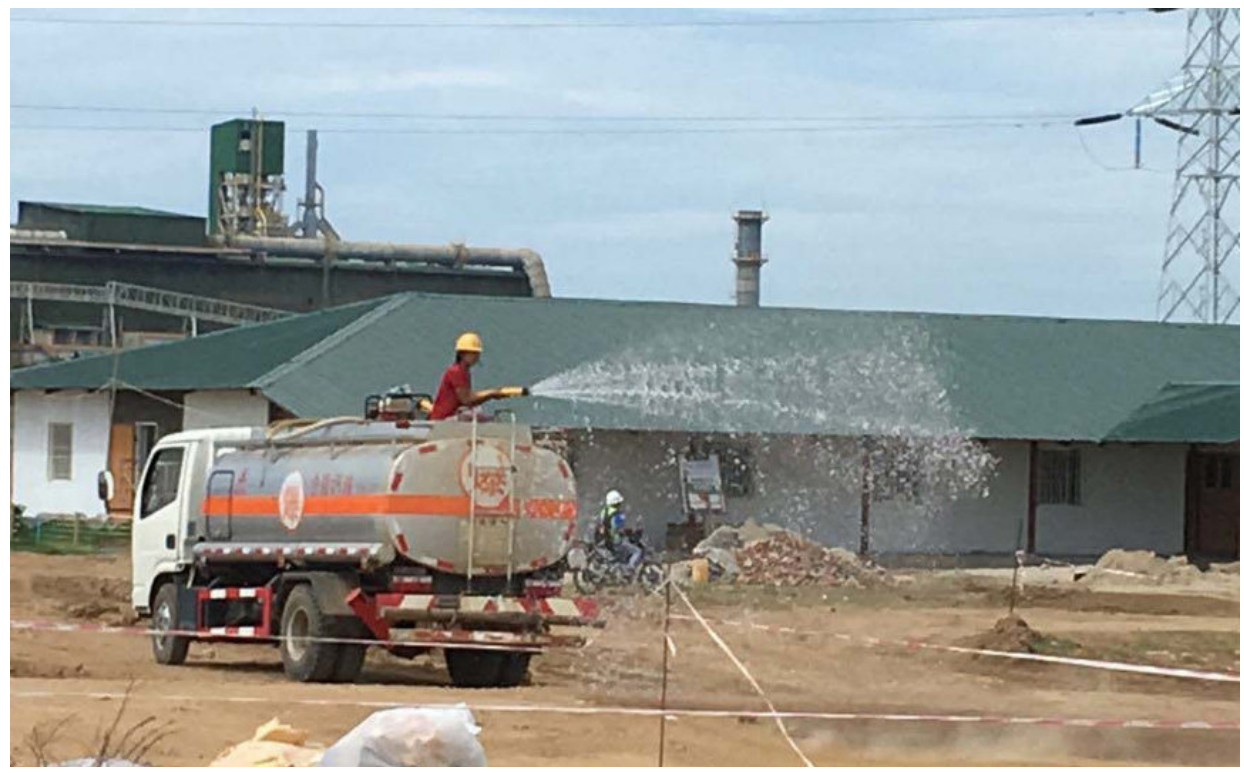
Photo 7: Dust suppression on site roads
