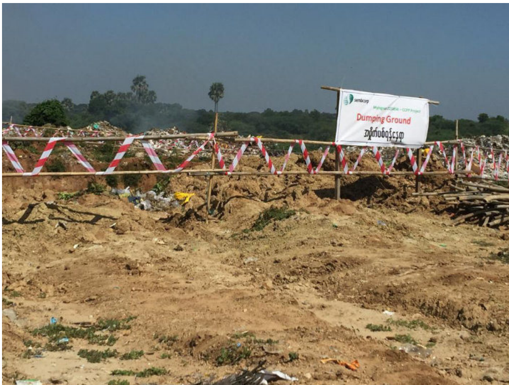
Photo 31: Newly demarcated project area at landfill site
