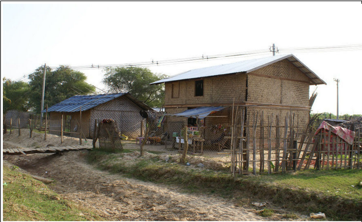
Photo 44: Old and new shops along the river water supply pipeline
