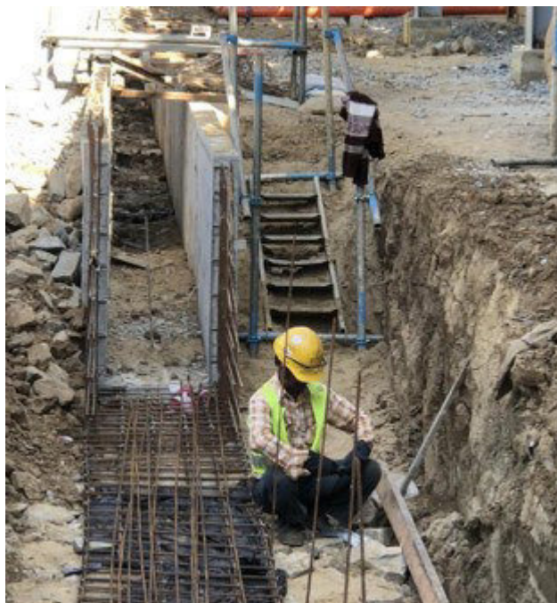
Photo 33: Safe access added to trench
