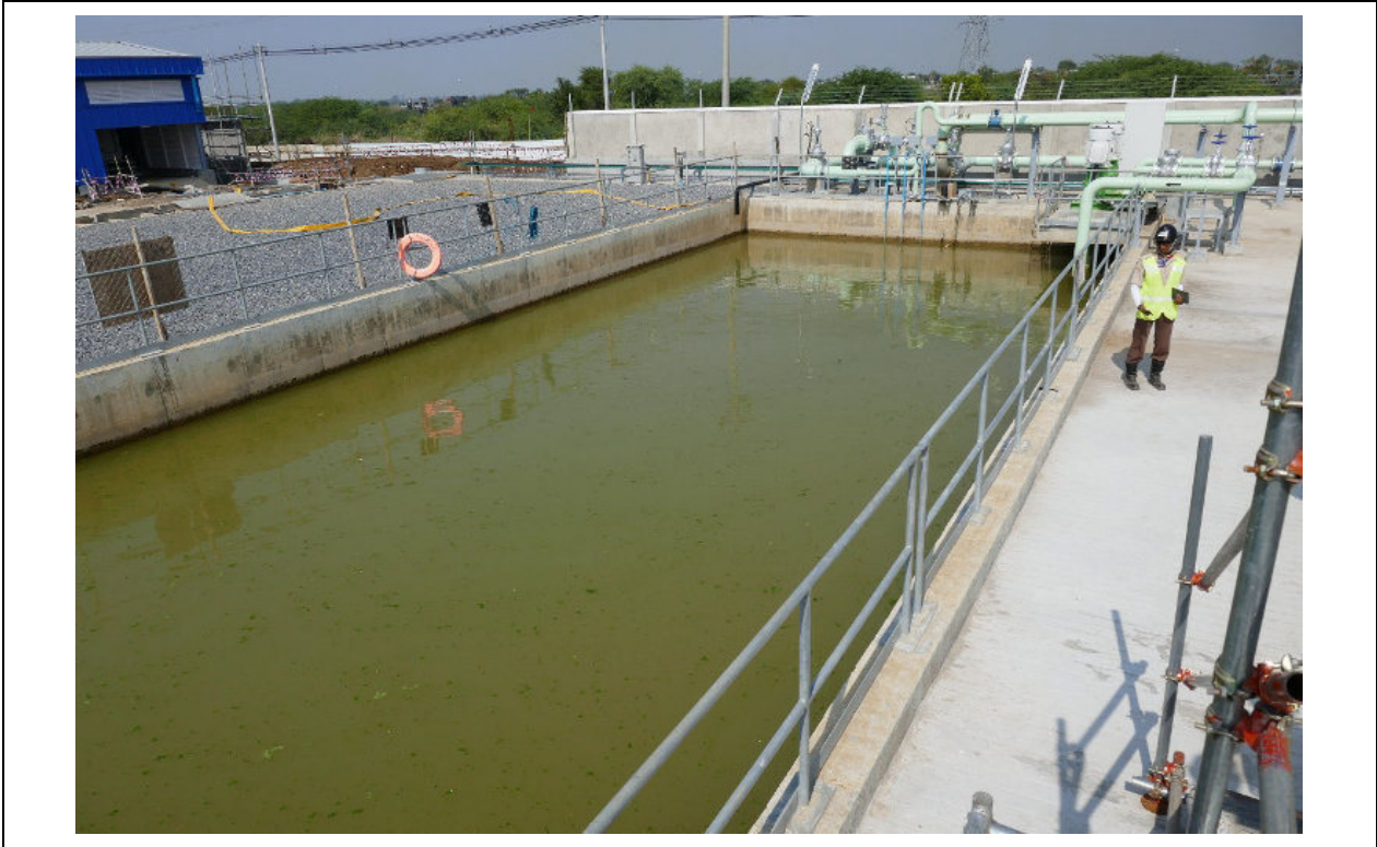
Photo 20: Central monitoring basin
