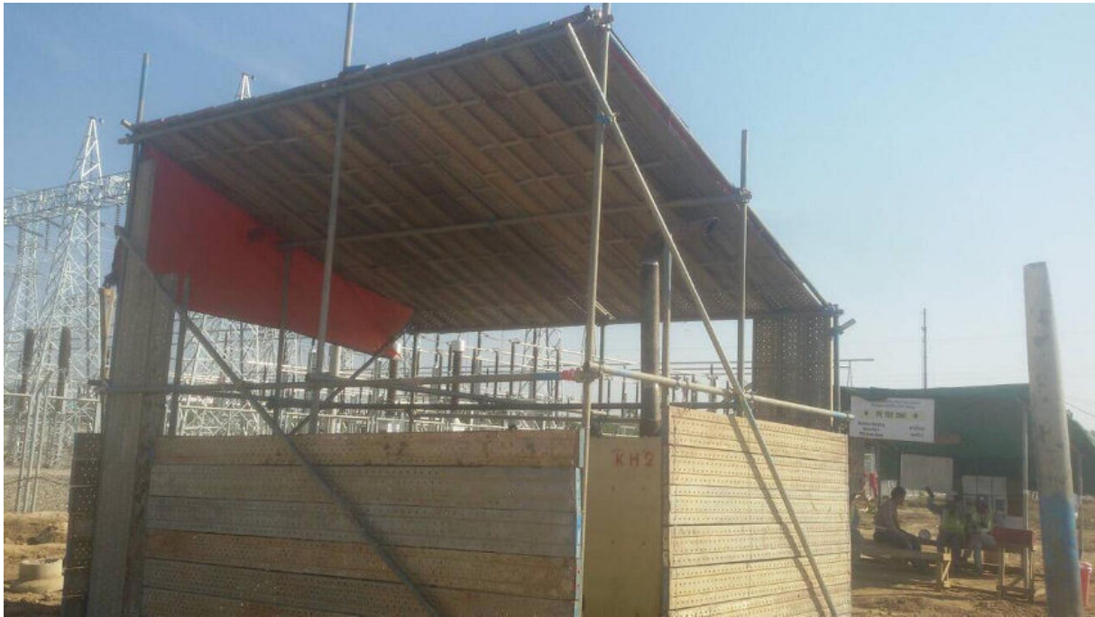
Photo 27: Roof over generator replaced immediately after site visit
