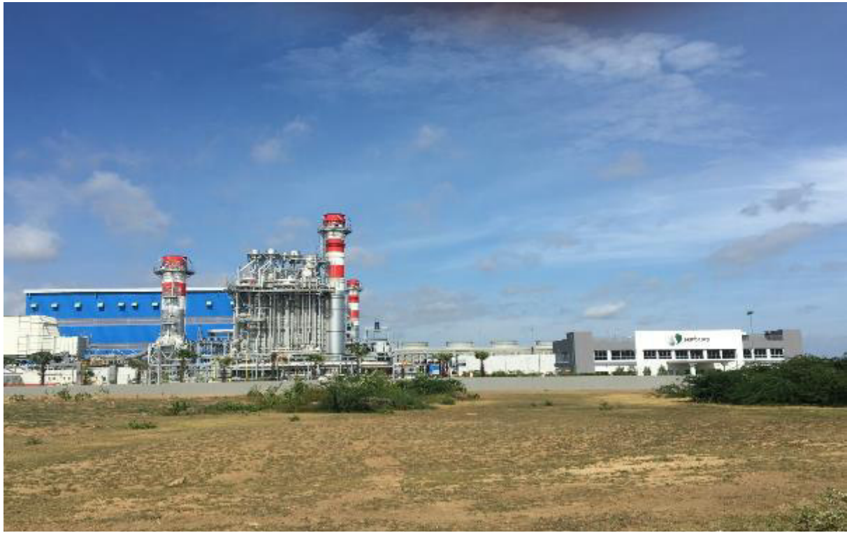
Photo 1: View of the Myingyan CCGT Plant as of August 2018.
