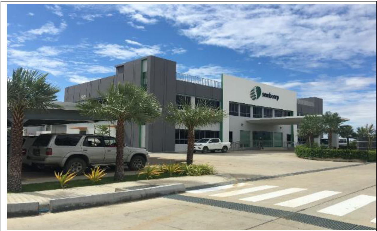
Photo 2: Completed administration building
