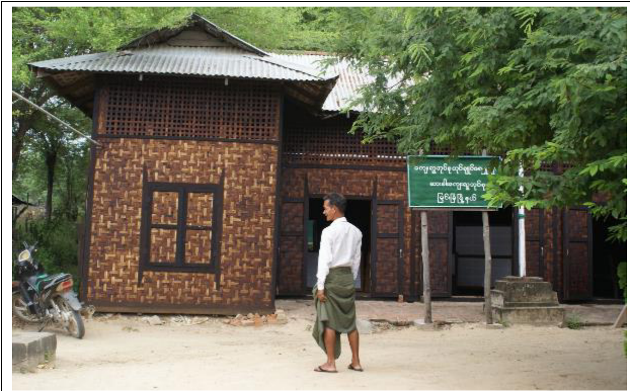
Photo 36: Sa Khar Village: Village Head and the Rebuilt GAD Office, a Sembcorp/PCo CDP Project
