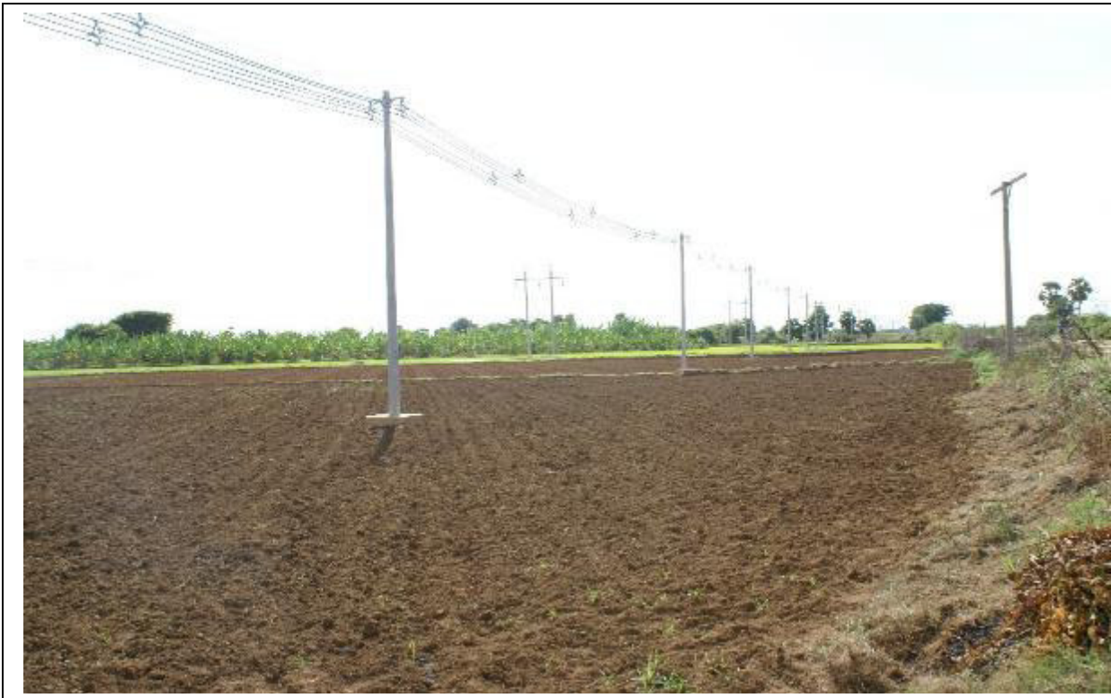
Photo 50: Field prepared for planting new crops along the buried river water supply pipeline
