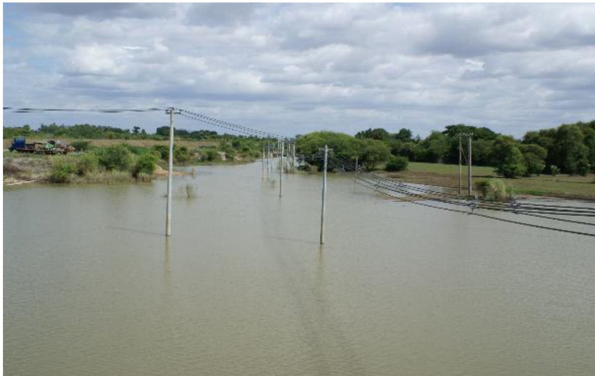
Photo 47: Seasonal flooding along the buried river water supply pipeline and power poles, facing towards the Myingyan power plant
