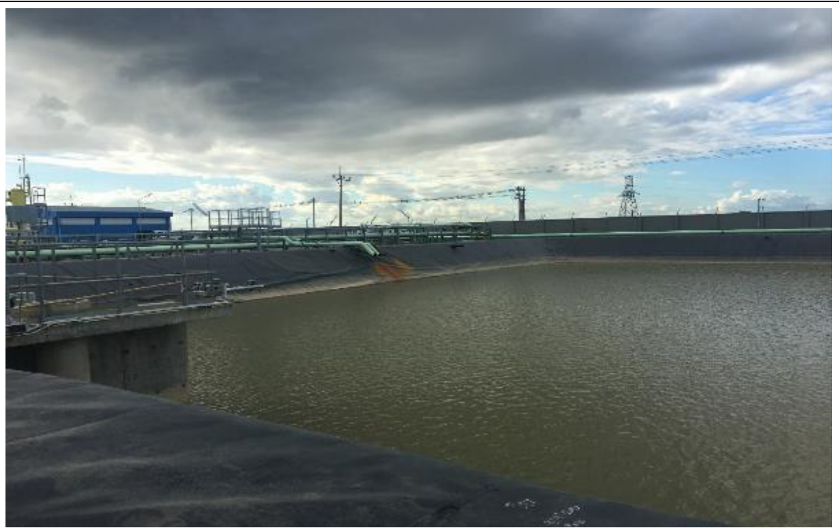
Photo 4: River water storage reservoir
