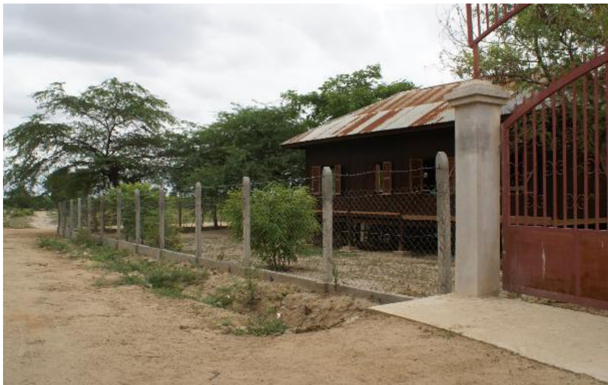
Photo 39: Sa Khar Village: Fence around the primary school, a Sembcorp/PCo CDP project
