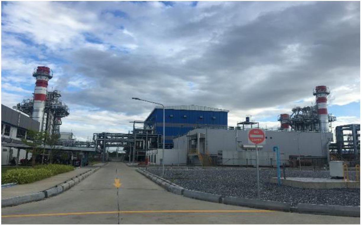
Photo 3: View of the two gas turbines
