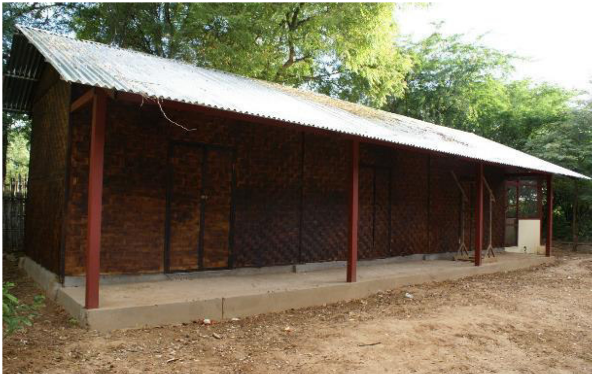
Photo 28: Nyaung Kan Village: Teachers' newly constructed living quarters, a Sembcorp/PCo CDP Project
