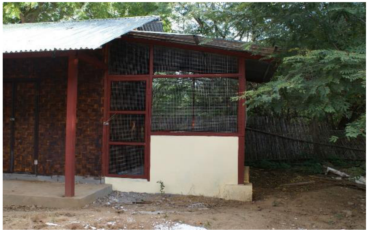
Photo 30: Nyaung Kan Village: Teachers' newly constructed kitchen, a Sembcorp/PCo CDP Project
