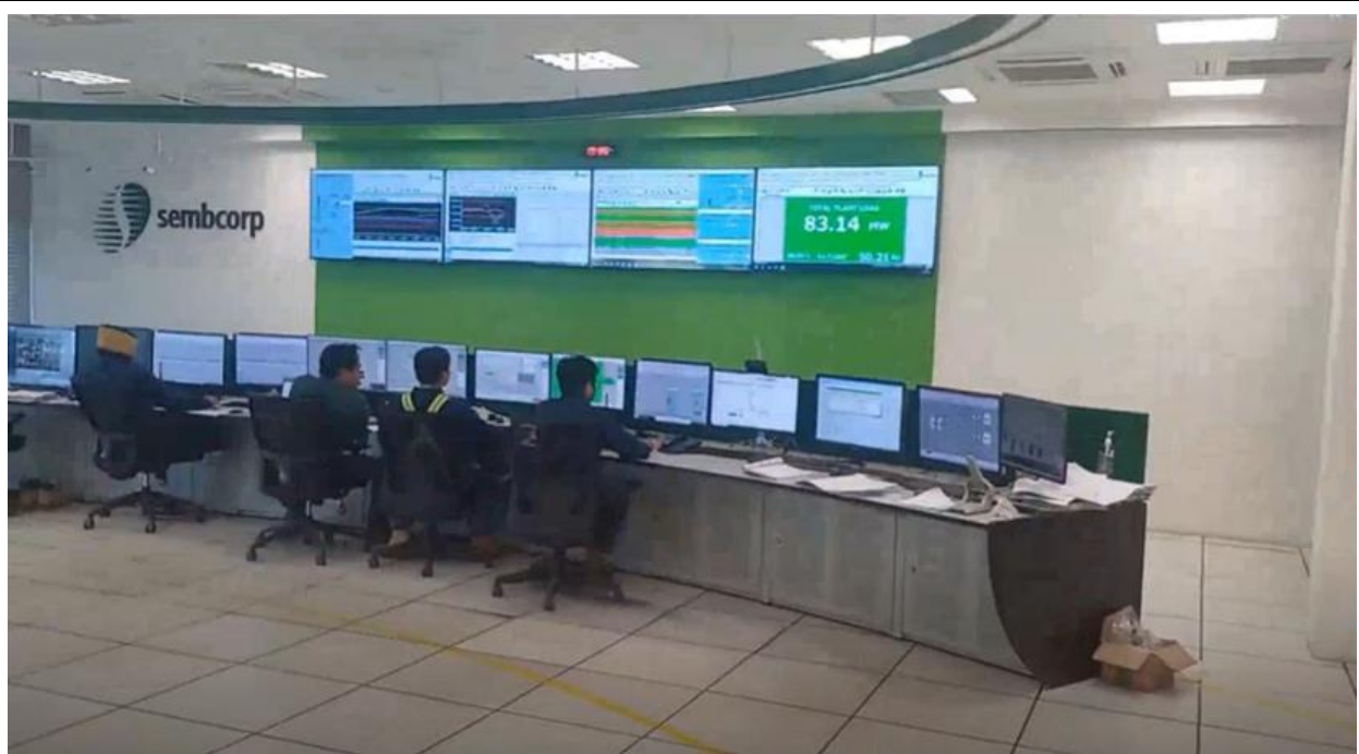
Photo 2: Plant Control Room with Continuous Operations Monitoring System within the main administration building (Photo taken from video during January 2025 Site Visit)
