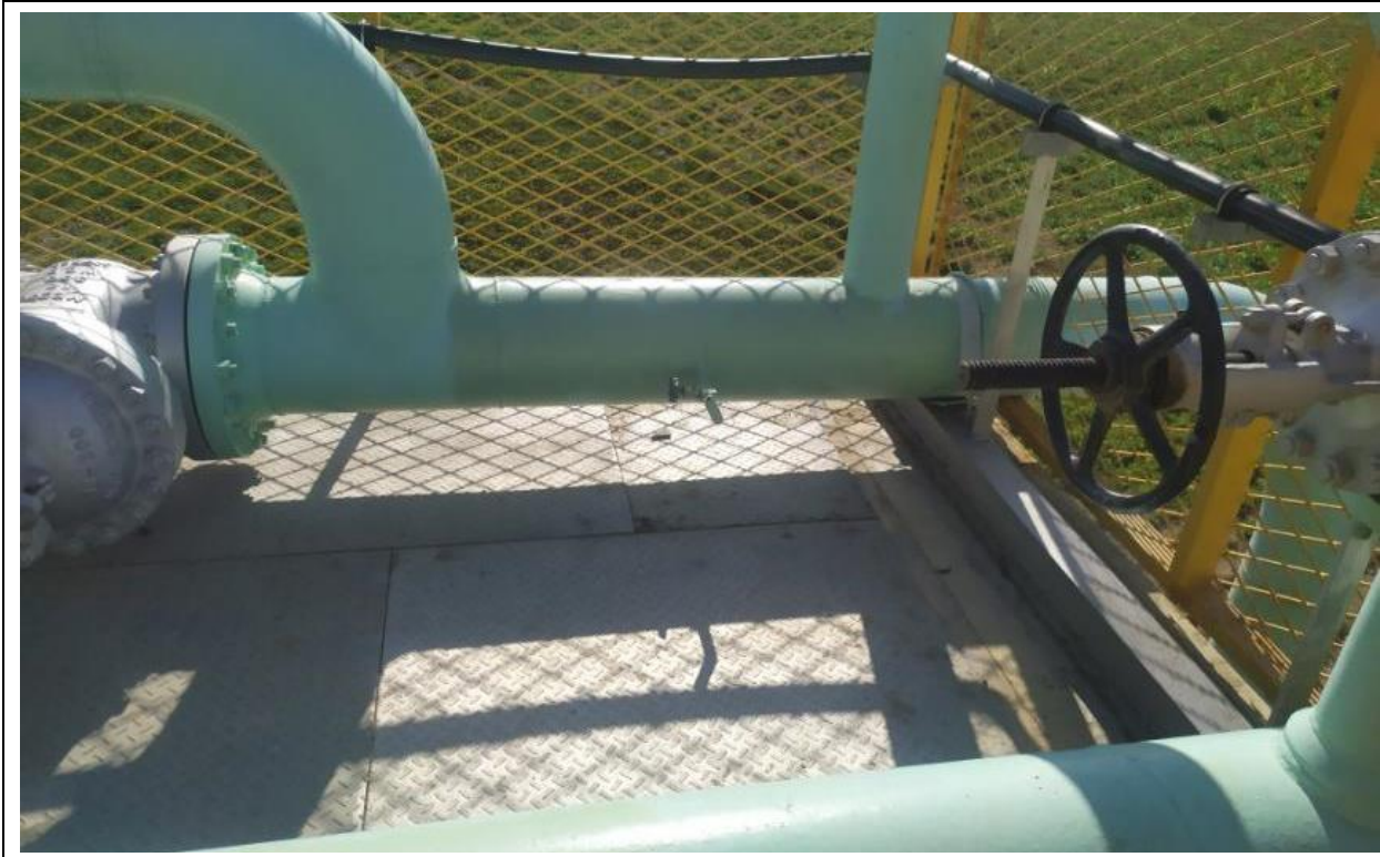
Photo 11: Designated water sampling location from the discharge pipeline (Photo provided by SMPC, January 2022 Site Visit)
