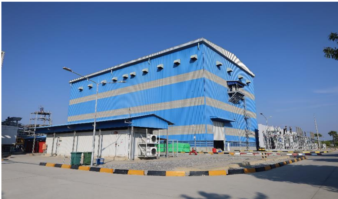
Photo 4: Steam Turbine Building (Photo provided during January 2025 Site Visit)
