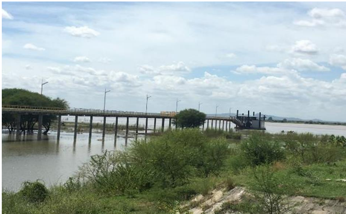
Photo 8: Overview of the river water supply pipeline and pumping station (December 2019 Site Visit)
