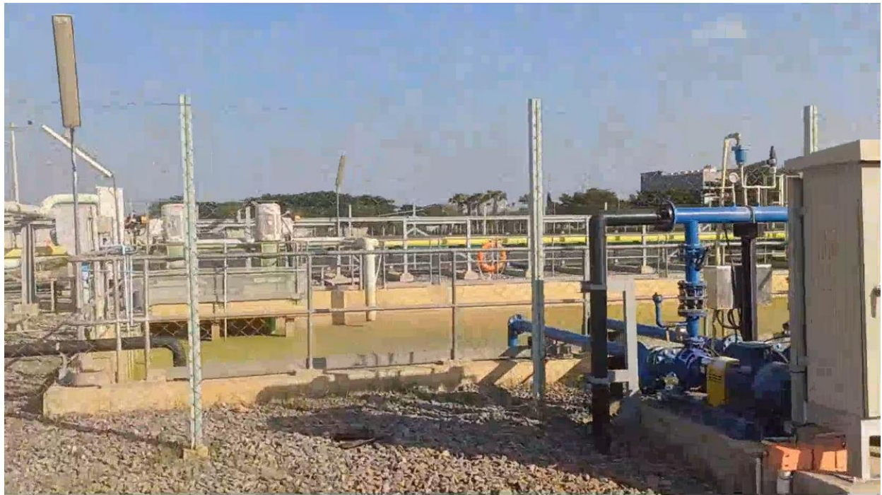
Photo 7: Central Monitoring Basin (Photo taken from video during January 2025 Site Visit)
