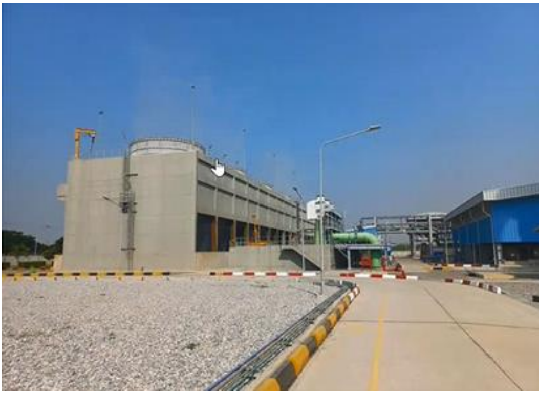
Photo 41: Cooling Tower (Photo taken from video provided for January 2023 Site Visit)
