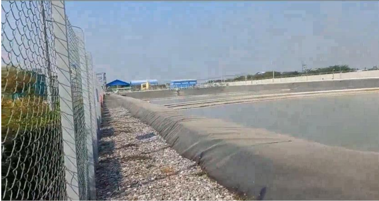
Photo 23: Raw Water Pond of water storage reservoir (Photo taken from video shared during January 2023 Site Visit)
