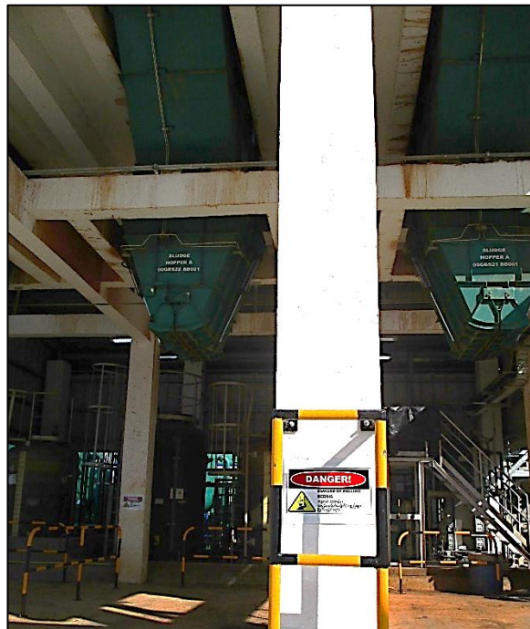
Photo 13: Sludge hoppers for collection of sludge from the water treatment plant (December 2019 Site Visit)
