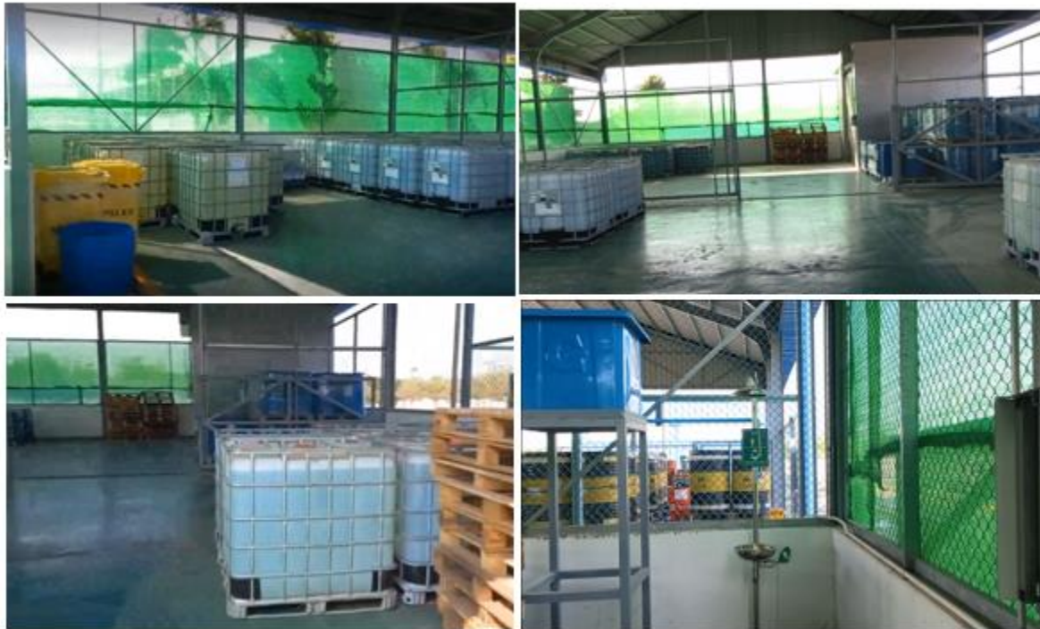
Photo 37: Chemical Storage Area with eyewash and emergency spill kits (Photos taken from video provided for January 2023 Site Visit)
