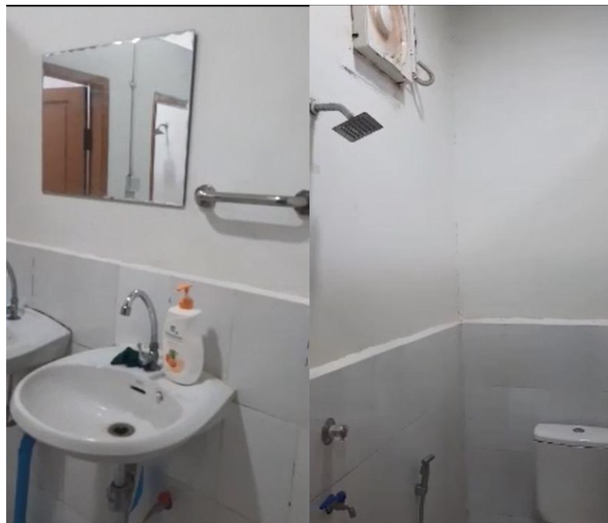
Photo 50: Male bathroom at Safe House 1 (Photos taken from video provided for January 2023 Site Visit)
