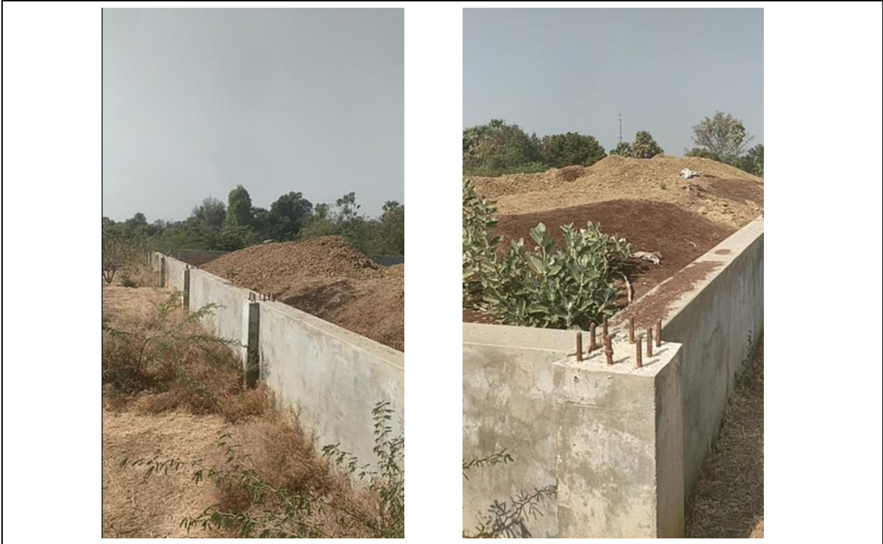
Photo 33: Off-site sludge storage facility owned and operated by OK Service for sludge from the water treatment plant (Photos taken from video provided for January 2023 Site Visit)
