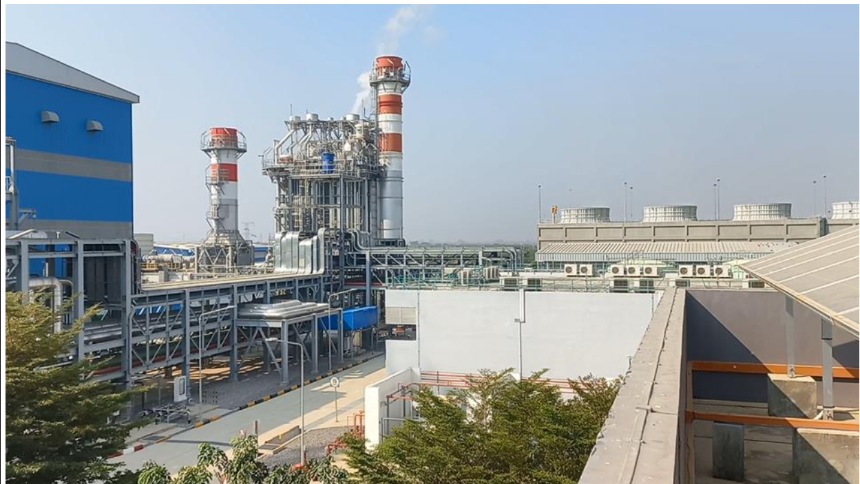
Photo 5: View of the Myingyan CCGT Power Plant from Administration Building rooftop (Photo taken from video provided during January 2023 Site Visit)
