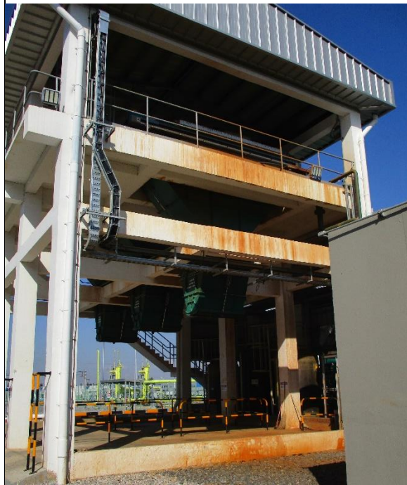
Photo 13: Sludge hoppers for collection of sludge from the water treatment plant (December 2019 Site Visit)
