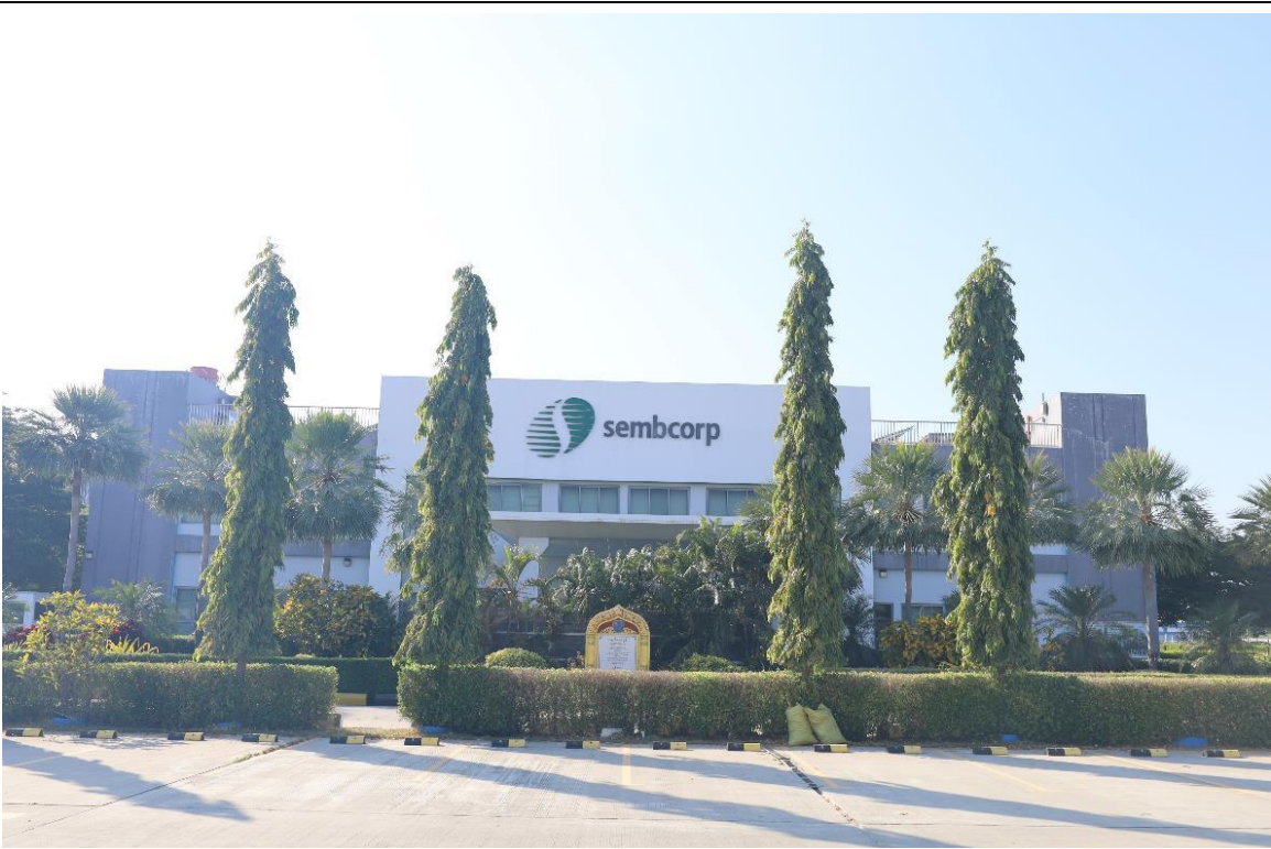
Photo 2: View of the Administration Building (Photo provided during January 2025 Site Visit)
