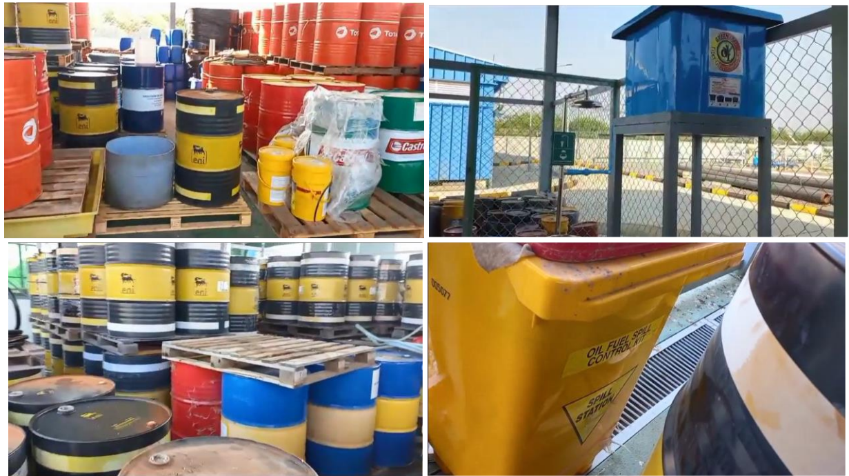
Photo 29: Inside Lube Oil Shelter with eyewash and oil fuel spill control kit (Photos taken from video provided for January 2023 Site Visit)
