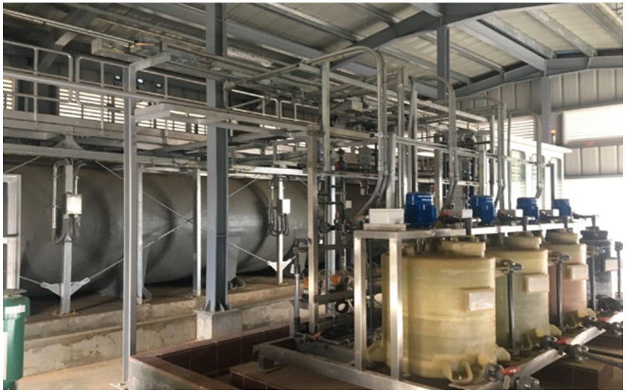
Photo 11: All sanitary wastewater from the Myingyan CCGT Plant is routed to the sanitary wastewater treatment plant
