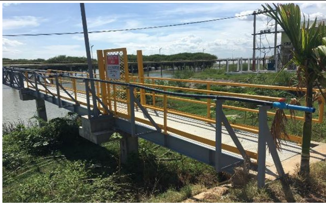
Photo 14: Entrance leading to the river water supply pumping station
