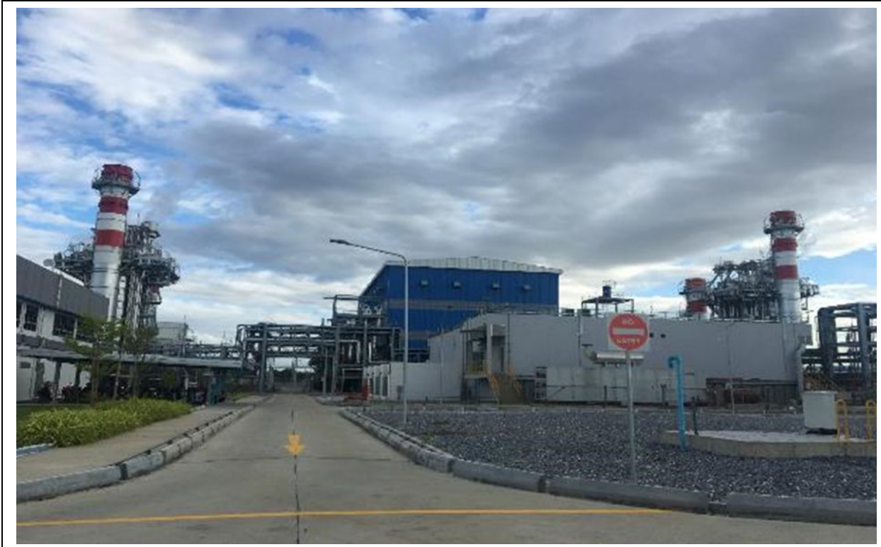
Photo 5: View of the two gas turbines
