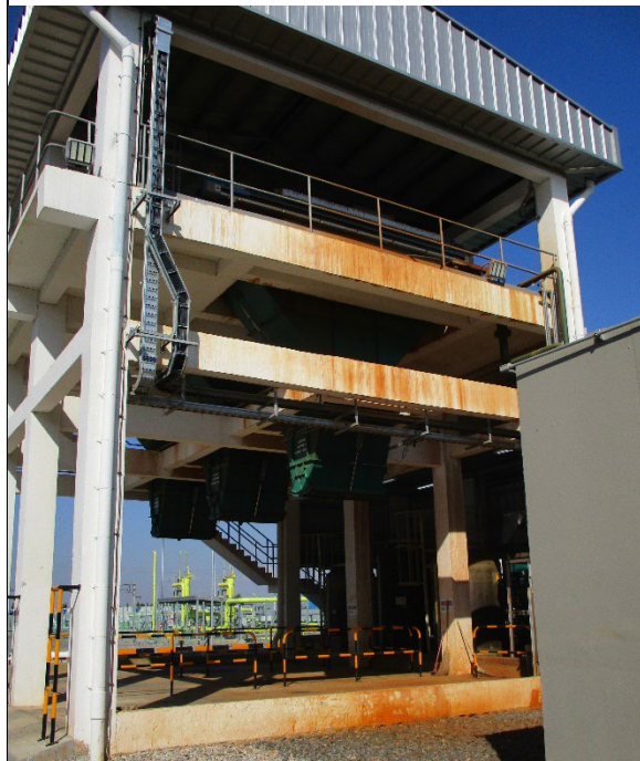
Photo 7: Sludge from the water treatment plant is collected at three (3) sludge hoppers and disposed by a licensed waste contractor.
