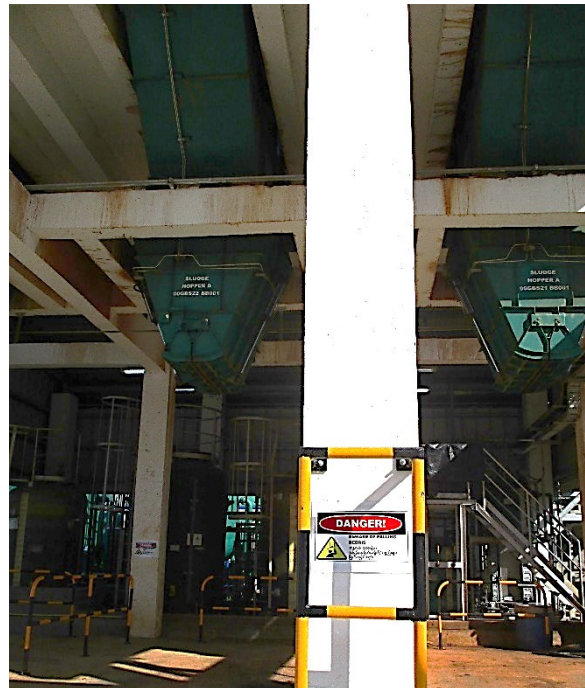
Photo 7: Sludge from the water treatment plant is collected at three (3) sludge hoppers and disposed by a licensed waste contractor.
