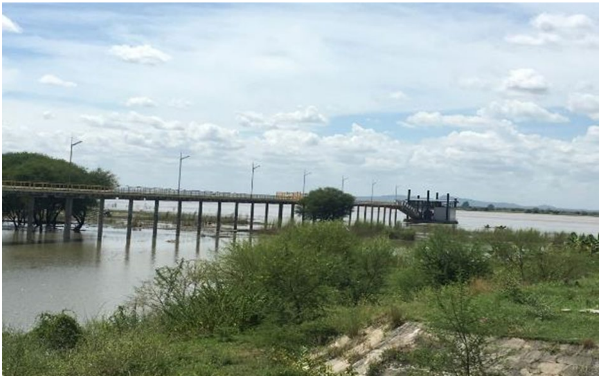
Photo 15: Overview of the river water supply pipeline and pumping station
