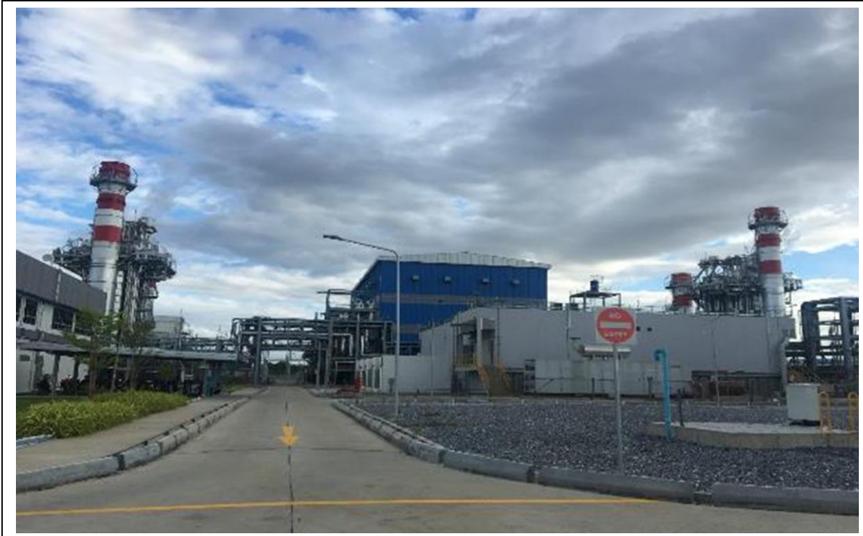
Photo 5: View of the two gas turbines (December 2019)
