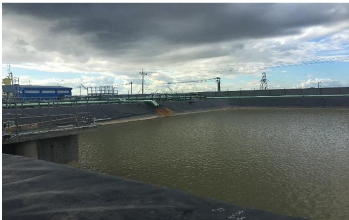
Photo 6: River water storage reservoir (December 2019)
