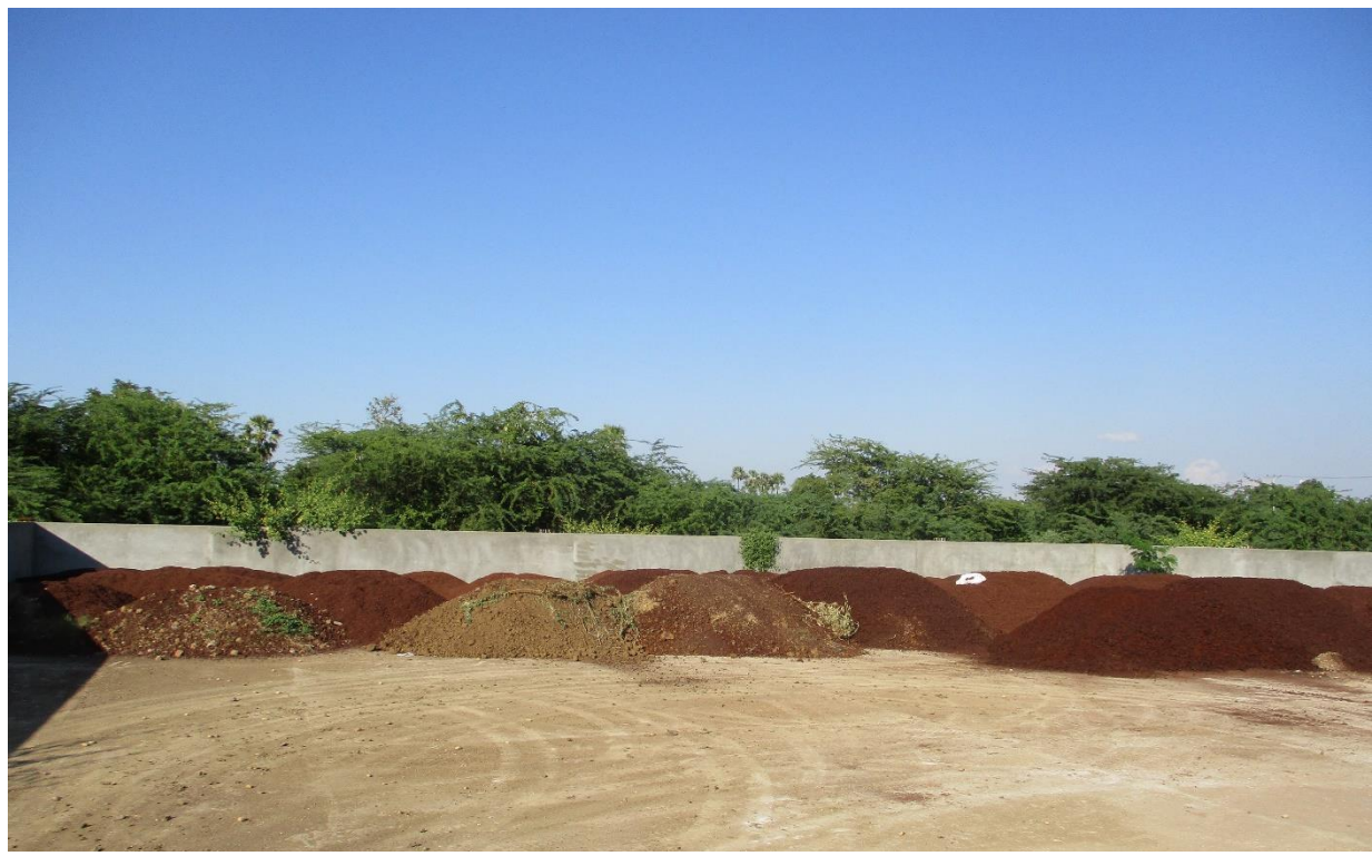
Photo 13: Off-site storage area owned and operated by OK Service for sludge from the water treatment plant (December 2019)
