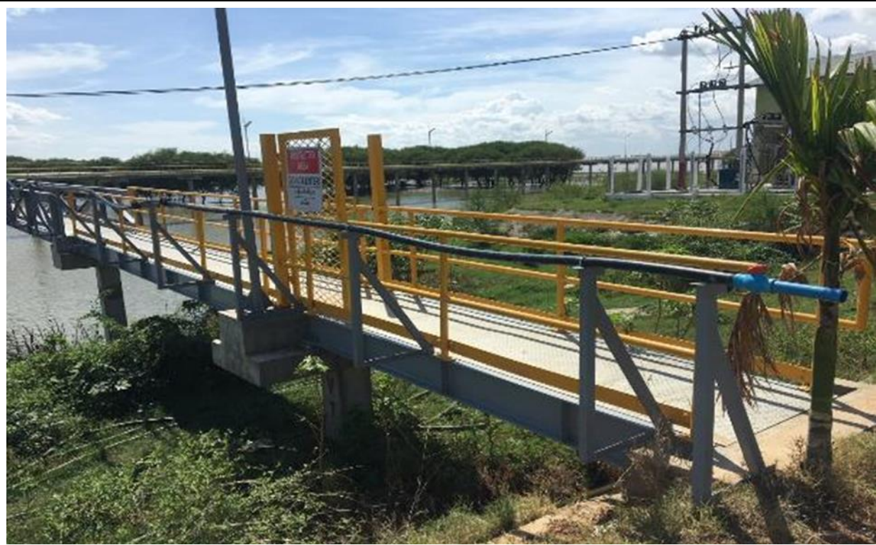
Photo 14: Entrance leading to the river water supply pumping station (December 2019)
