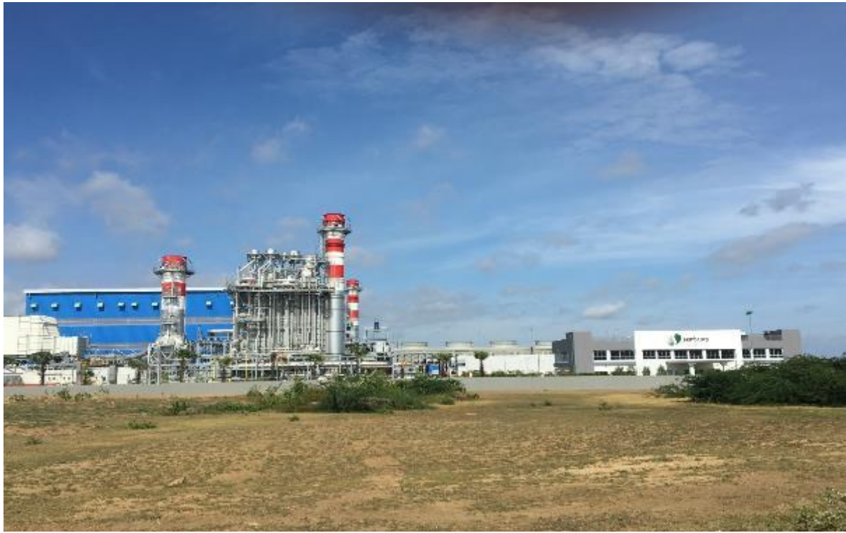
Photo 1: View of the Myingyan CCGT Plant (December 2019)
