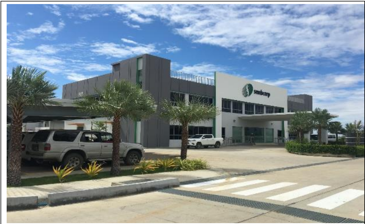
Photo 2: View of the Administration Building (December 2019)
