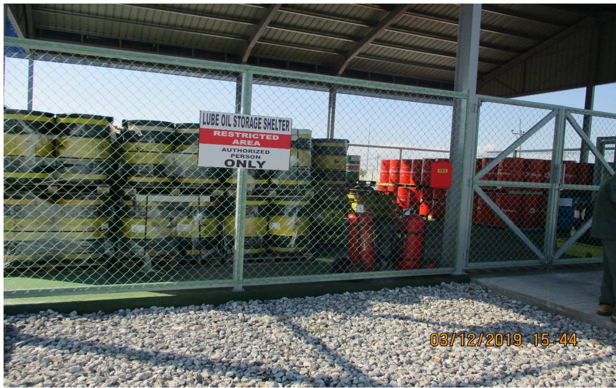
Photo 8: Lubricant oil storage area (December 2019)
