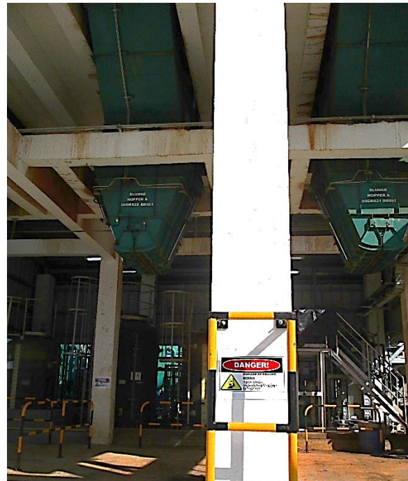
Photo 7: Sludge hoppers for collection of sludge from the water treatment plant (December 2019)
