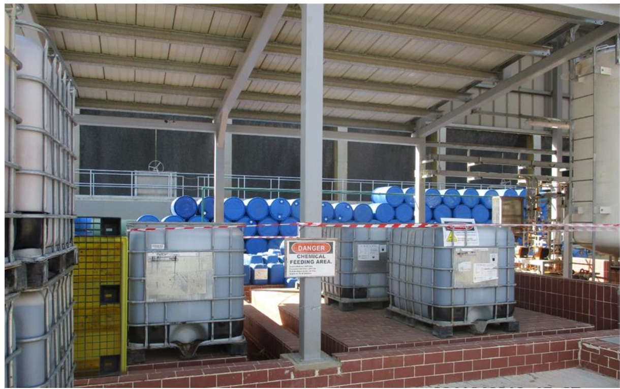
Photo 10: Chemical feeding area (December 2019)
