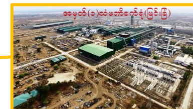
No.1 Steel Mill, Myingyan
