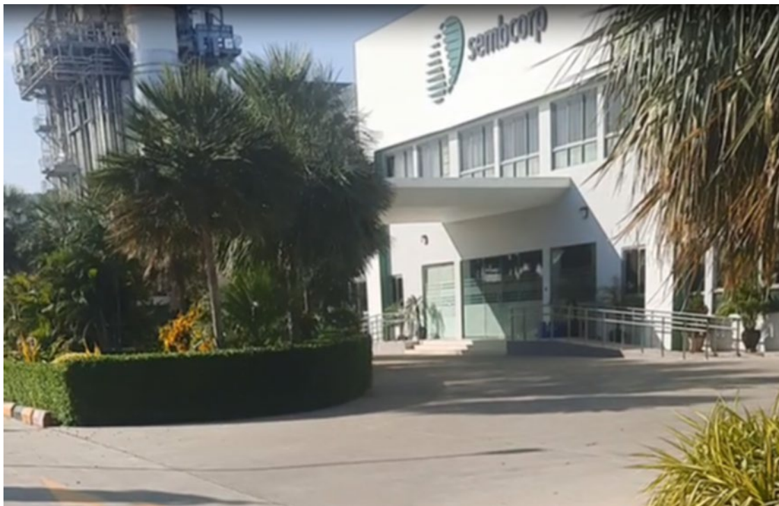
Photo 2: View of the Administration Building (Photo taken from live video during February 2022 Audit)
