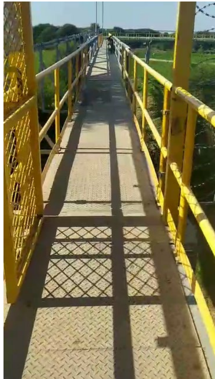
Photo 20: Entrance leading to the river water supply pumping station (Photo taken from video provided by SMPC, January 2022)
