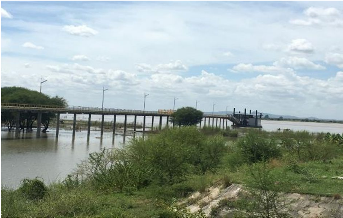
Photo 3: Overview of the river water supply pipeline and pumping station (December 2019)
