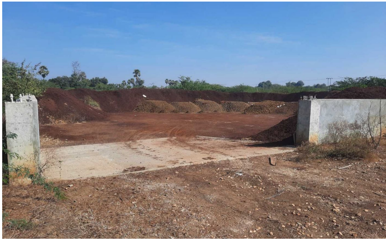
Photo 19: Off-site storage area owned and operated by OK Service for sludge from the water treatment plant (Photo provided by SMPC, January 2022)
