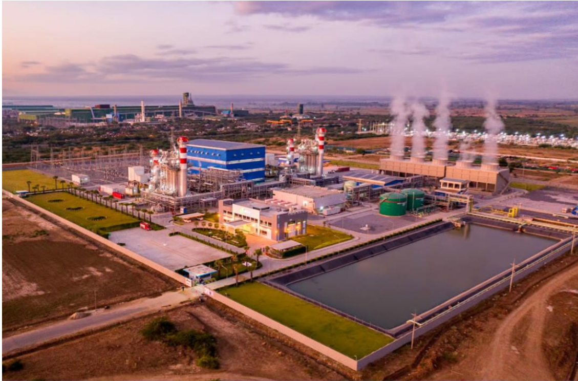
Figure 3: Project Aerial (Photo from Sembcorp)
