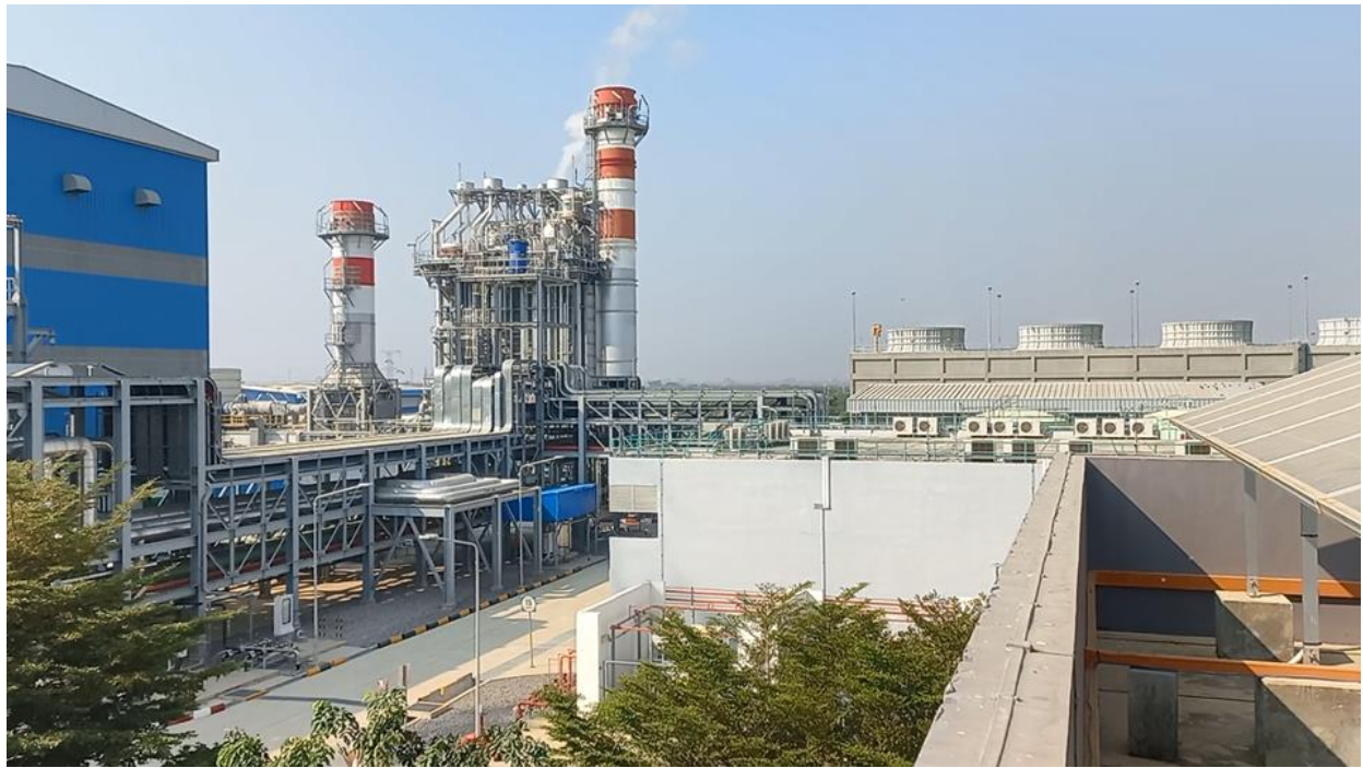
Photo 1: View of the Myingyan CCGT Power Plant from Administration Building rooftop (Photo taken from video provided during January 2023 audit)
