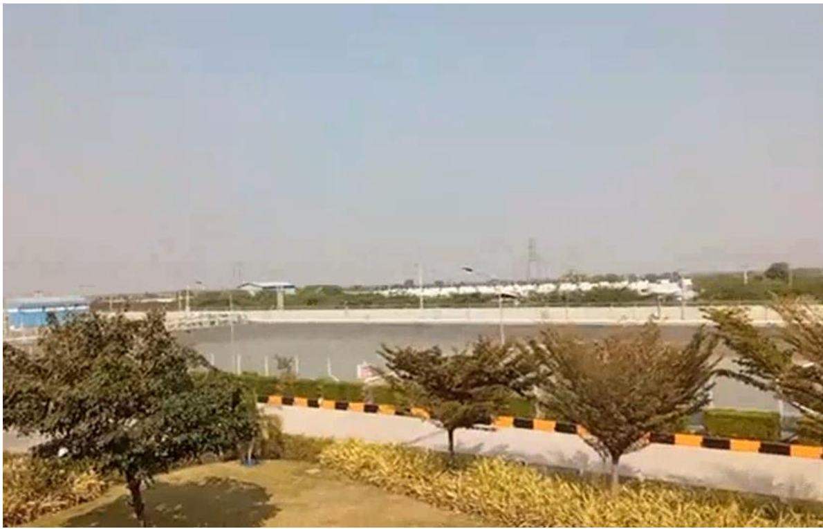
Photo 7: View of V Power and river water storage reservoir from office in administration building (Photo taken from live video during January 2023 audit)
