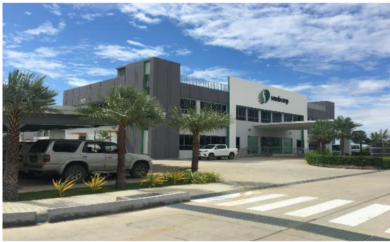
Photo 12: View of the Administration Building (December 2019)
