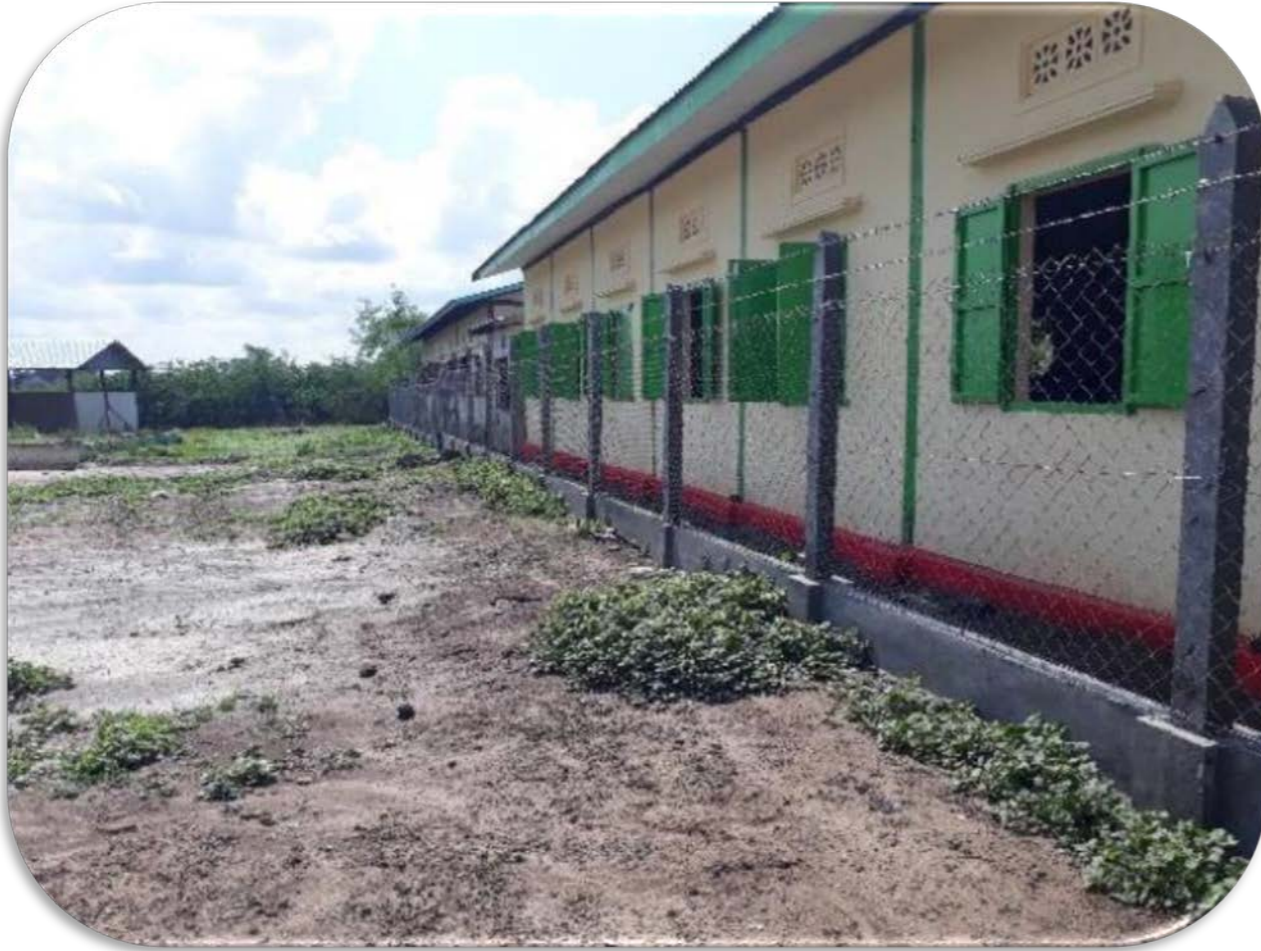
Newly Constructed the fence of the school compound
